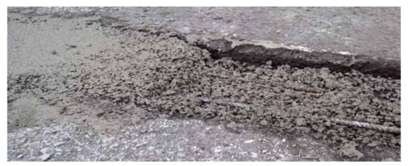
The Monopatch repair system has been derived from the ability to create a grouted macadam system mixed completely in the asphalt batching plant, having the freedom to be laid in one process (*see MonoConfalt*). Using unique asphalt and concrete techniques and traditional equipment thus makes it ideal for pothole repair.
